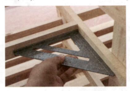
To check for square, we use a tool called a square. It is a right triangle (a triangle with a 90-degree angle) made from metal
