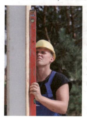
Checking to see if something is plumb is simple. Take a string and attach a weight to it. Attach the free end of the string to the top of the item you're checking, and let the weight pull the string down. Make sure the weight doesn't touch the ground. This string is plumb and can be used as a guide.
